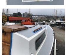
resealing the forehatch, sealing the windows and fitting new winch pads and hand rails, as well as fairing the keel.
