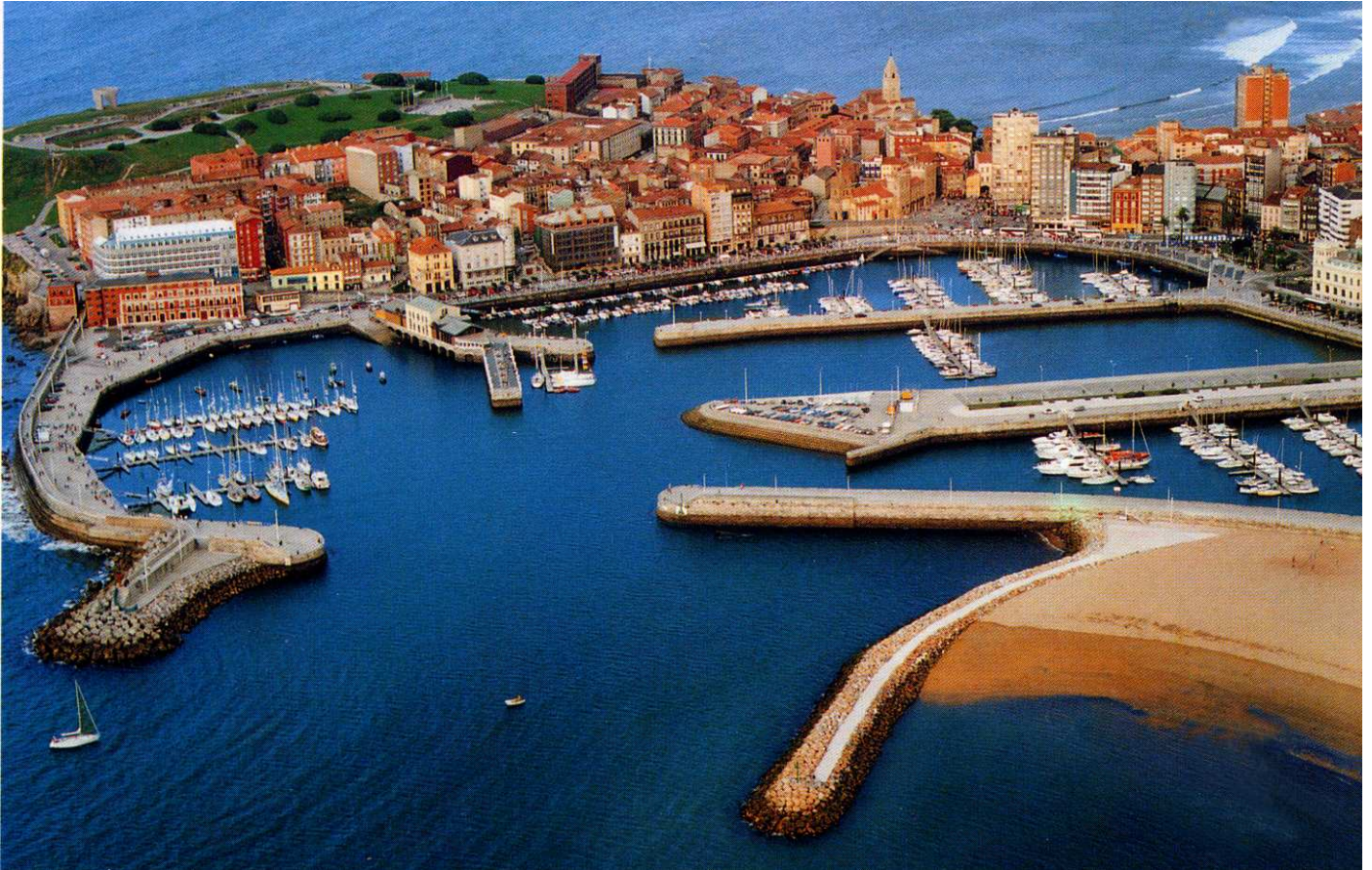
Gijón old harbour converted into a marina. This photo is quite old, the 3 basins to the right are now filled with yachts & motor boats. Of the pontoons to the left adjacent to the outer sea wall, the nearest 2 are for visitors, the far one for local small craft, the lifeguard’s boats etc.
